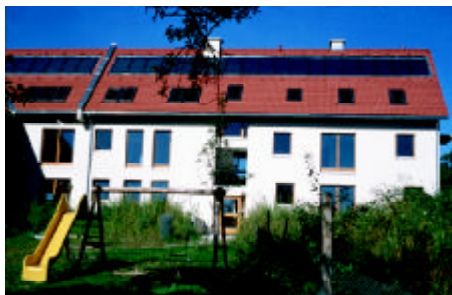
Contracting - Solaranlage Albersdorf
